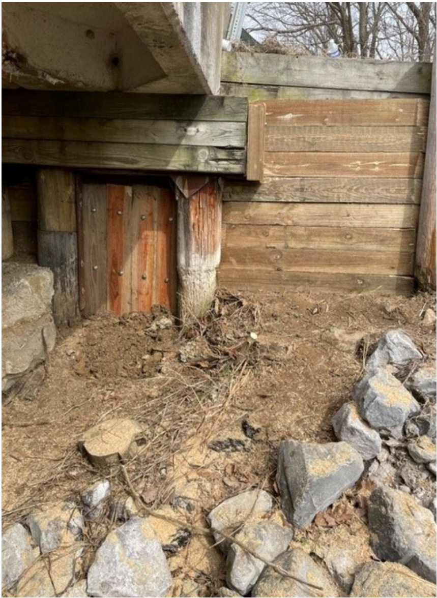
ABUTMENT #2 Right wingwall and Breastwall Repaired
