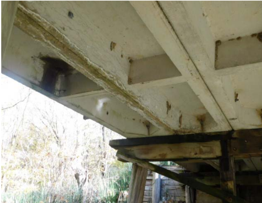
SPAN #2, SLAB "B" CRACKED
