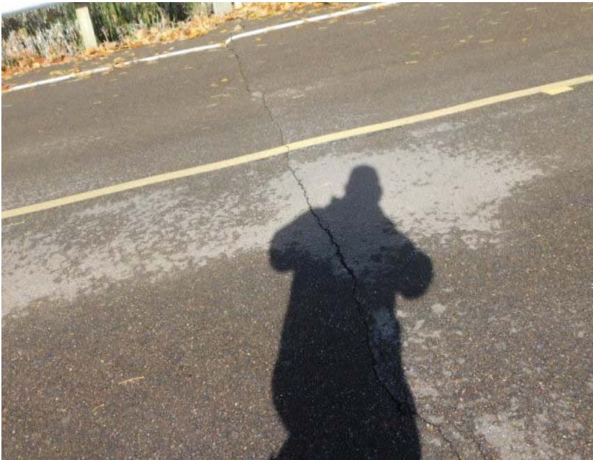
APPROACH #1 ASPHALT SETTLED
