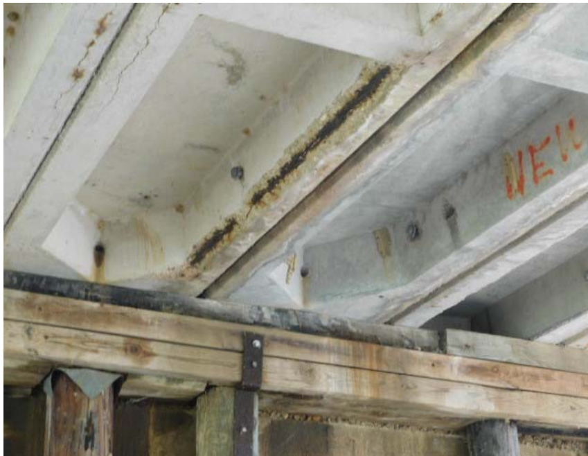
SPAN #3, SLAB "C" SPALLED TO STEEL
