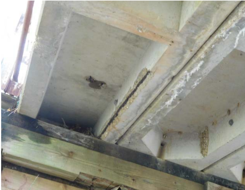
SPAN #3, SLAB "A" SPALLED TO STEEL
