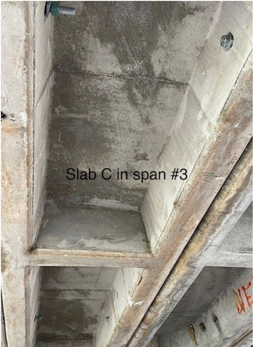
Span #3 Slab 'C' replaced
