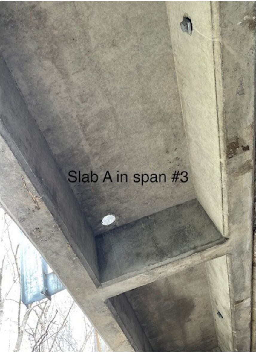
Span #3 Slab 'A' replaced
